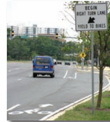
bicycle lane/pocket bike lane markings
